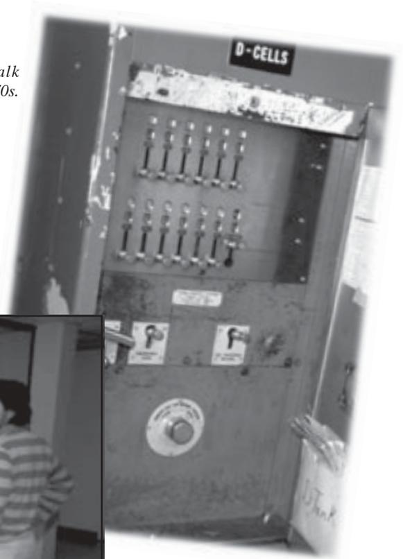
(Above) Control panel "D" Cells. (Note the hand crank to gang release all cells.)
